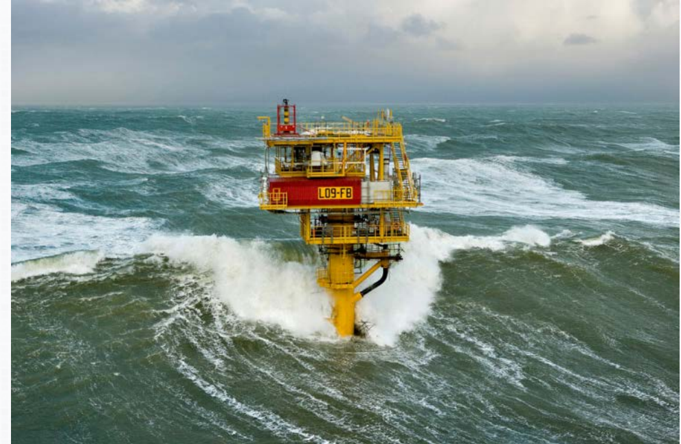
Breaking wave on a monopile offshore platform in shallow water (© www.flyingfocus.nl )
